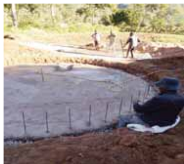
Construction of the water tank.
